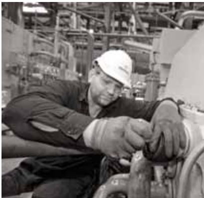
Mechanical Tradesperson Jeff Harbeck at Stanwell Power Station
