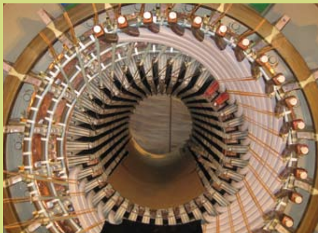
View of the end of the Unit 3 generator stator, showing a number of the new conductor bars installed.
