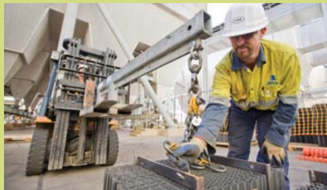
Workers preparing air heater baskets prior to installation.
