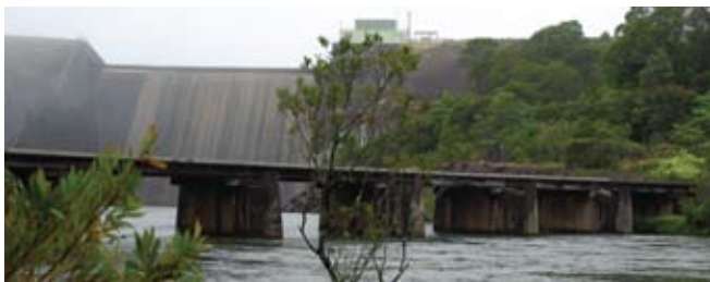
Koombooloomba Bridge before work commenced on the upgrade.
