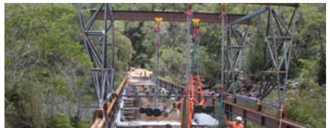
Removing the old timber decking.
