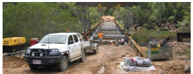
Using the gantry crane to install new precast concrete headstocks
