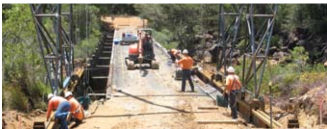
Installing the gantry crane for the Koombooloomba Bridge upgrade.
